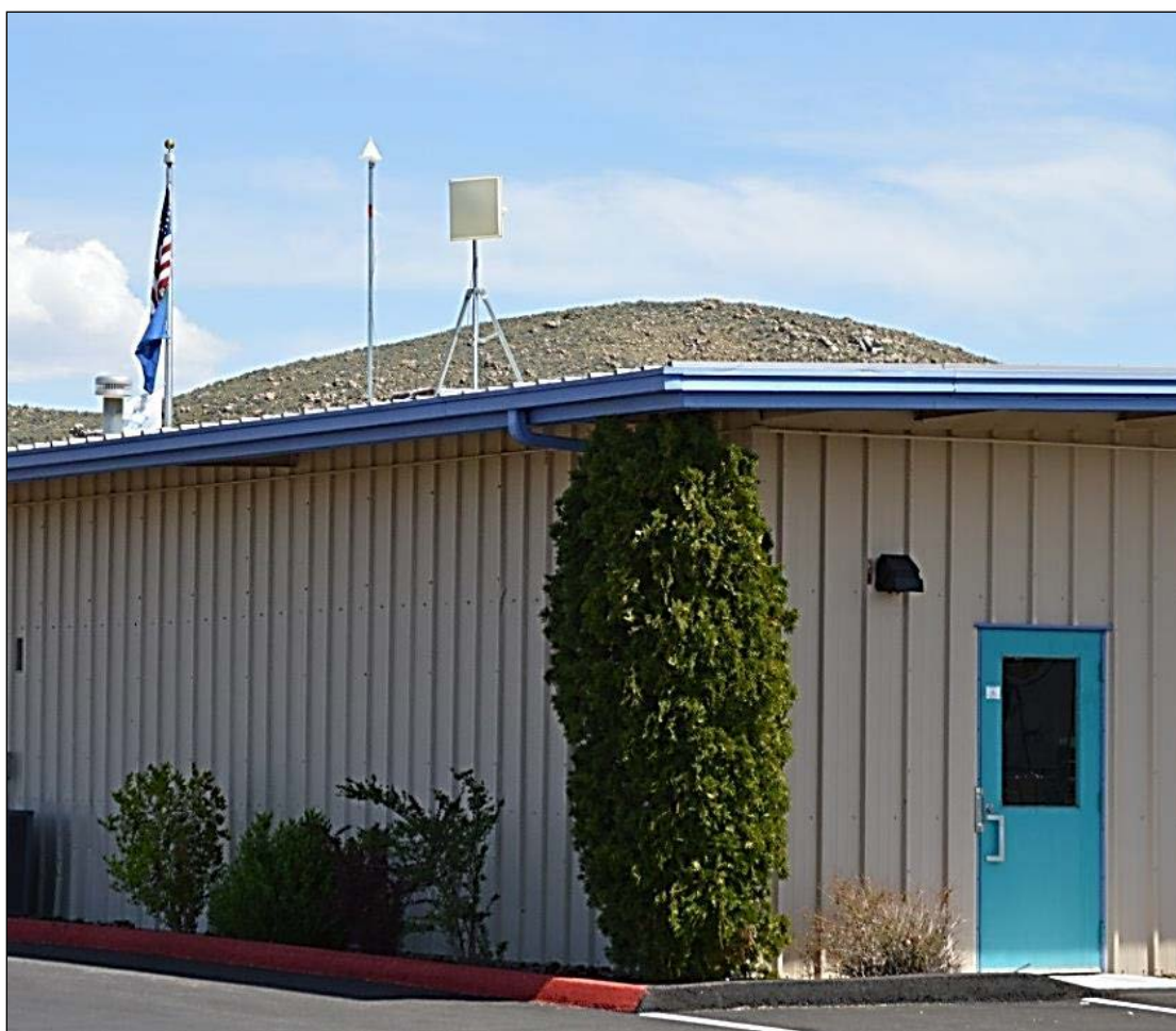
Figure 6 Lemmon Valley Monitoring Station
