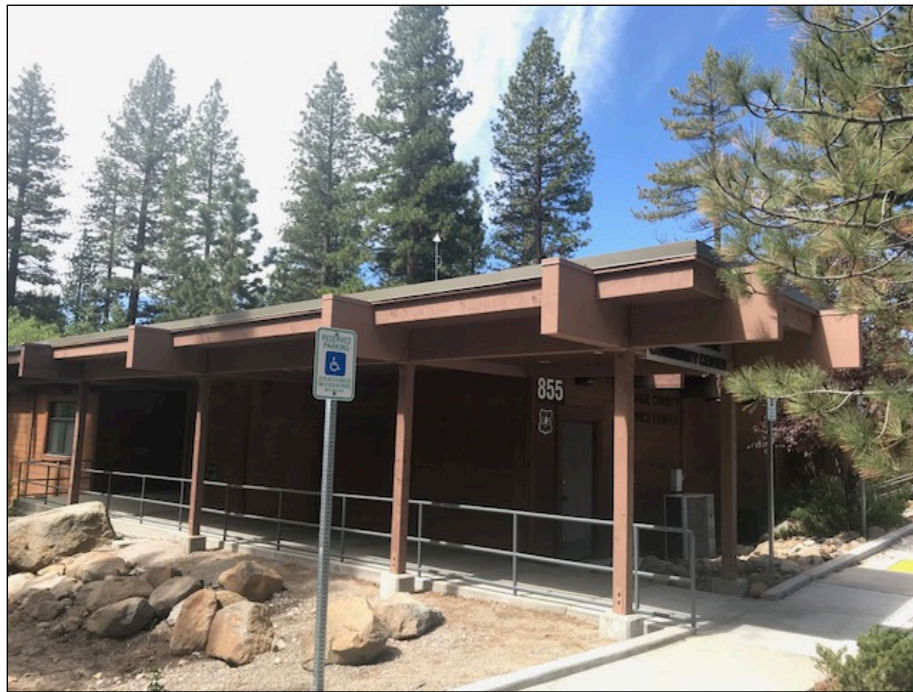
Figure 4 Incline Monitoring Station
