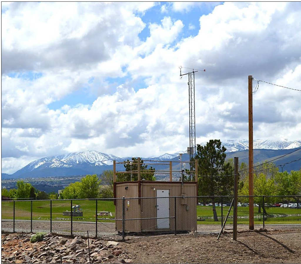
Figure 12 South Reno Monitoring Station
